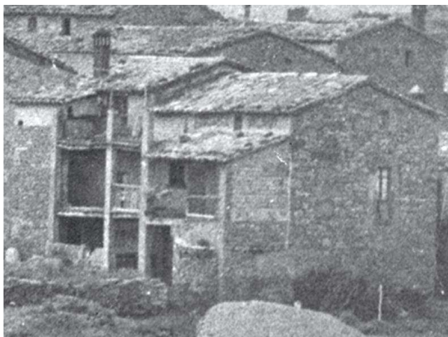
Vista general (c. 1960).
